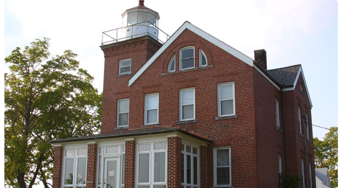
South Bass Island Lighthouse, now owned by The Ohio State University. Photo: Rene Sturgell · CC BY-SA 3.0 · Wikimedia Commons
